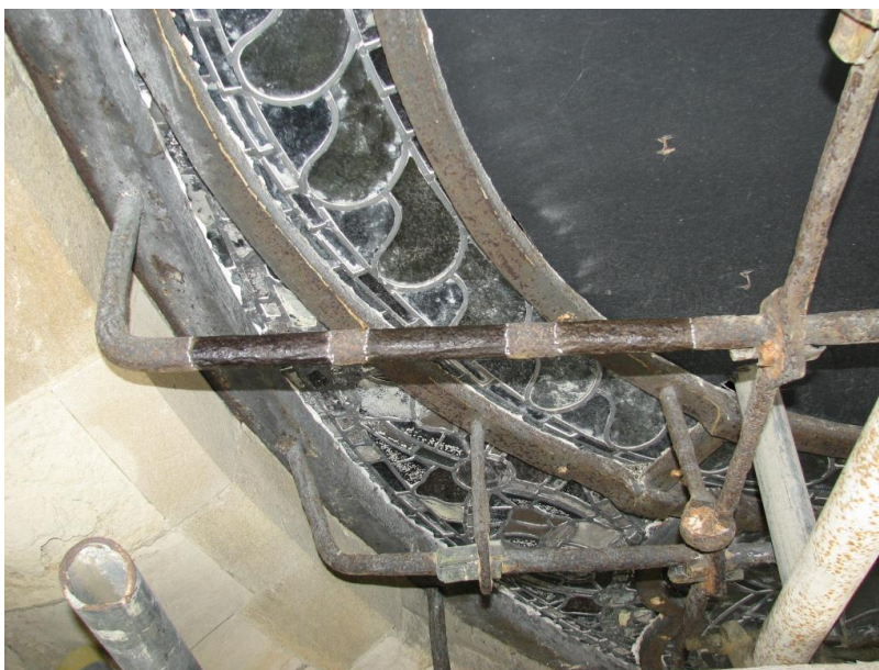
Fig.13: Cleaning and treatment trials on the metalwork
