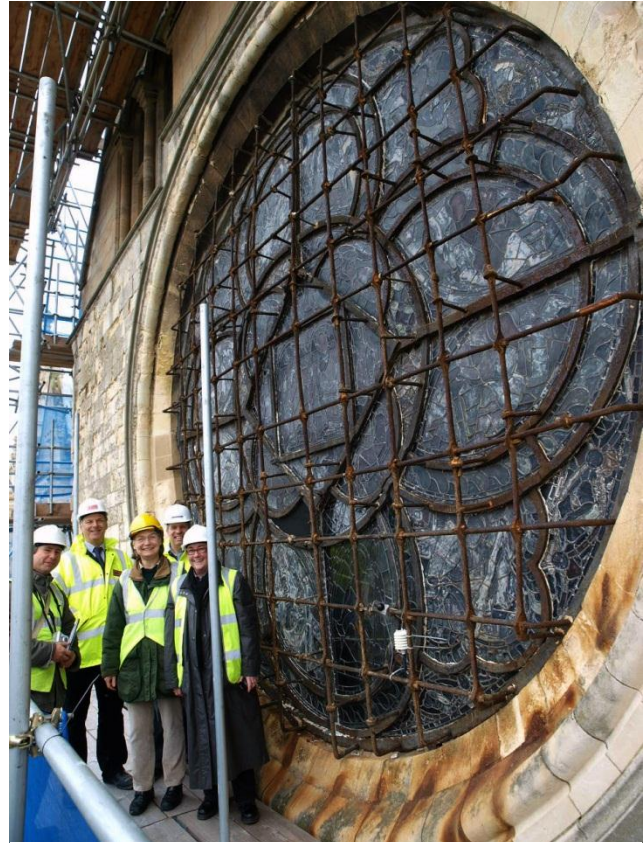
Fig.1: The exterior medieval ‘space frame’ on the South Oculus window
