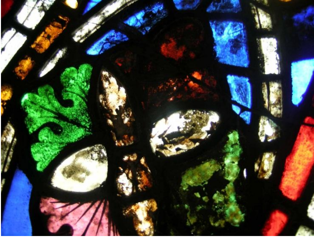
Fig.10: Medieval glass showing corrosion damage
